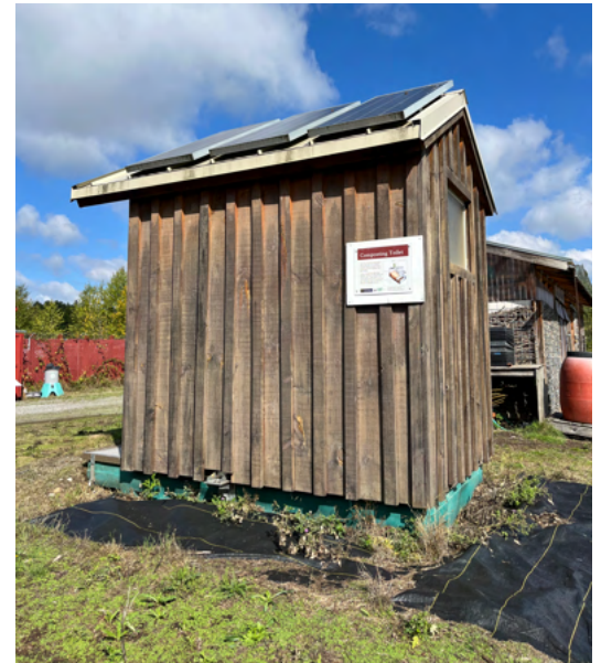
Signage helps to explain the compost toilet system at the UW Farm.
