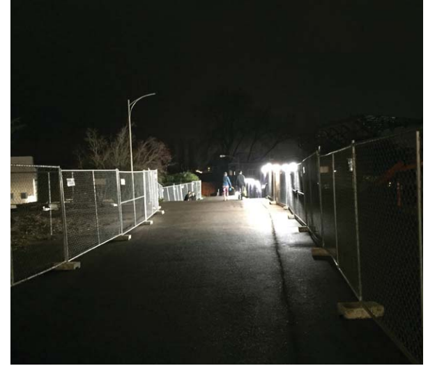
Figure 24. Temporary lighting on construction fence at site of the future Computer Science & Engineering building.
